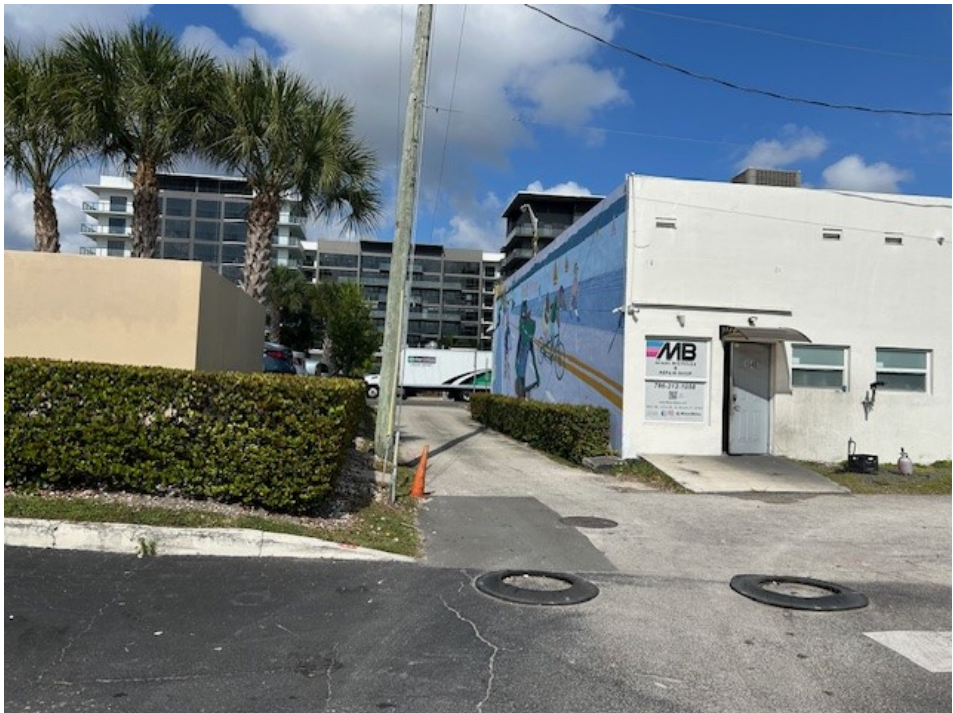
Site access from the north
